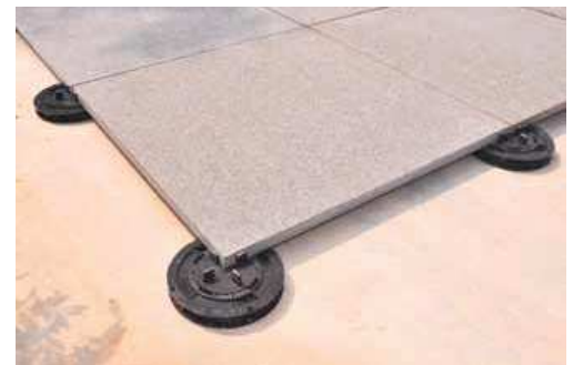
EAD providing support for porcelain pavers
