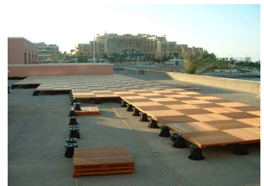
EAD providing support for timber decking
