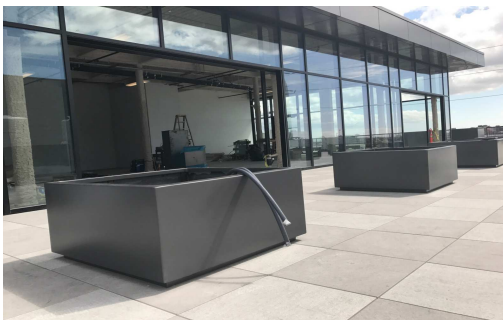
Coca Cola Bottling Plant Roofdeck Los Angeles, CA
