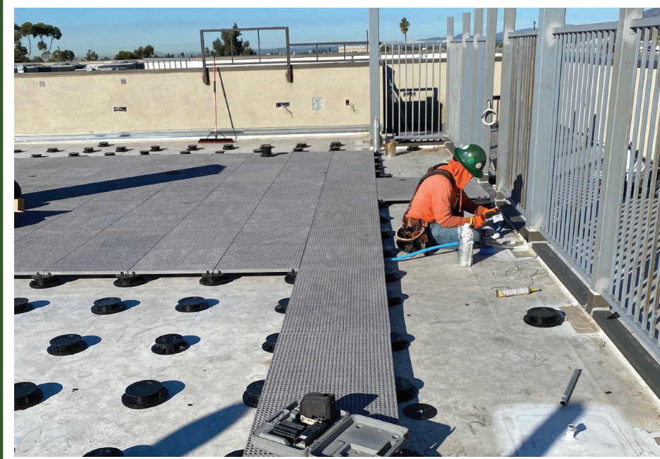
FRP grating with porcelain pavers on rubber Rise It fixed support pads
