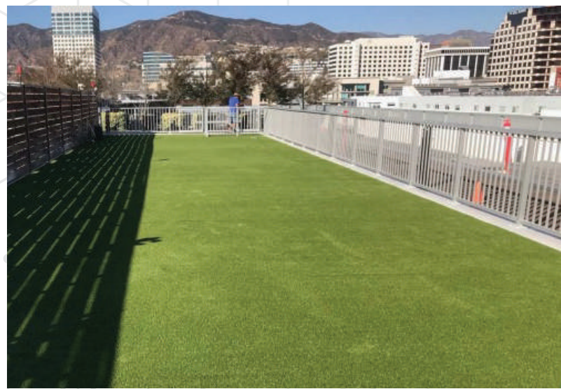
Turf installed on Roof Deck in Los Angeles
