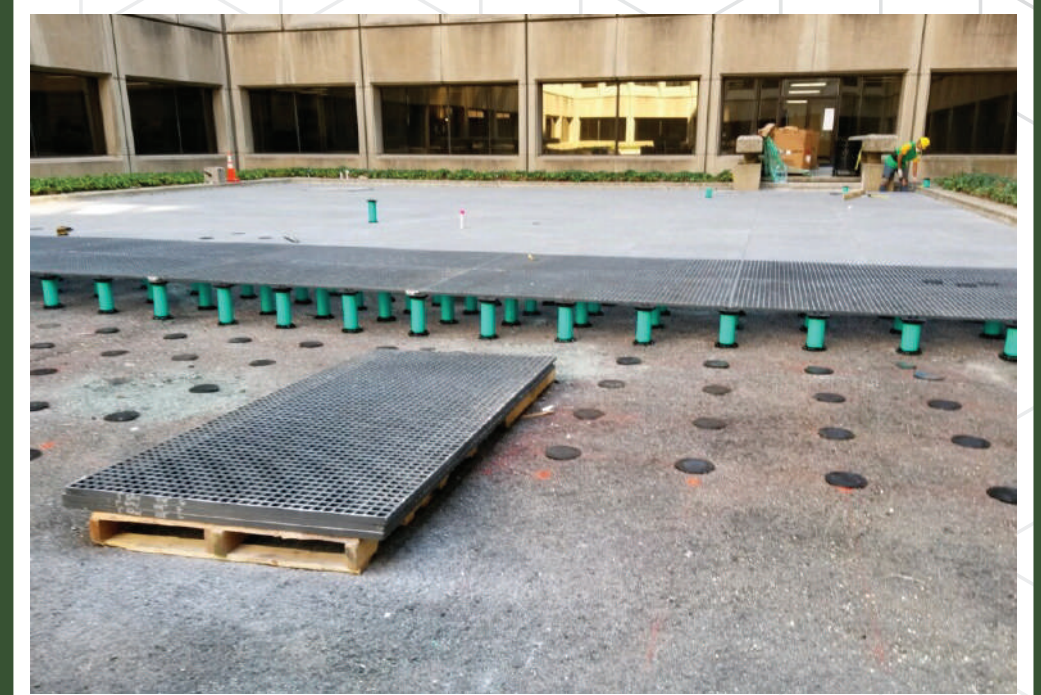
Deck Turf installed on foam block supports
