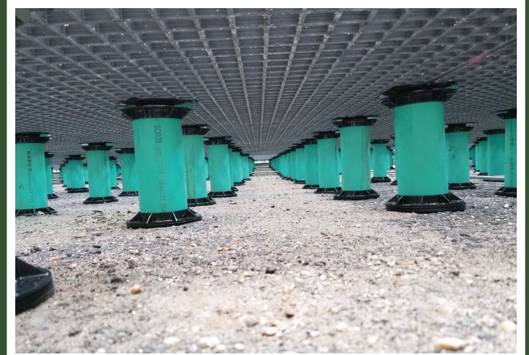
Plaza deck with porcelain pavers over FRP grating
