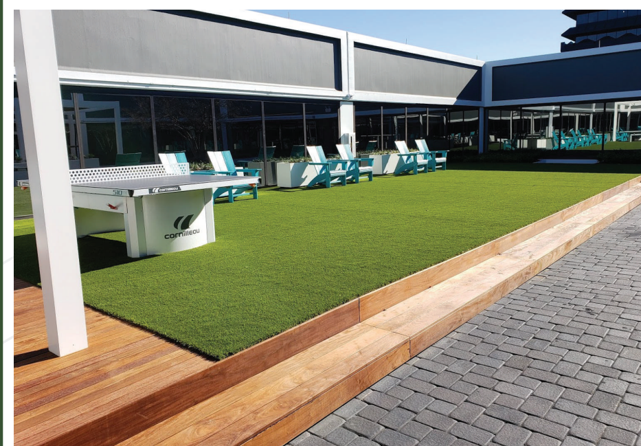
Project US Department of defense plaza deck porcelain paver on FRP grating
