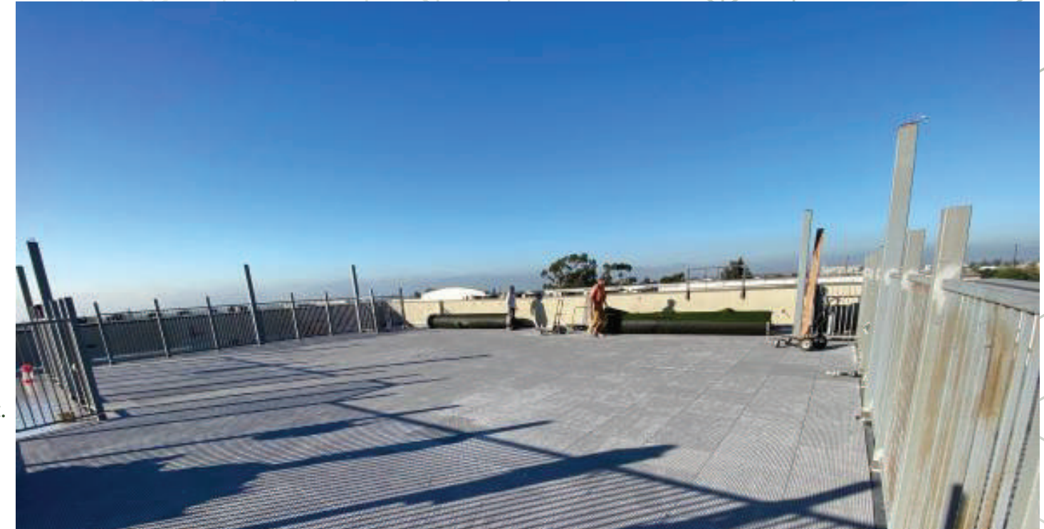
Completed FRP Deck Ready for Surface Material
